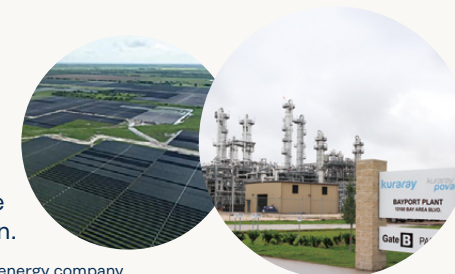
Left: Aktina Solar Power Plant (owned by Tokyo Gas America Ltd.) Right: Kuraray America's Bayport Plant
